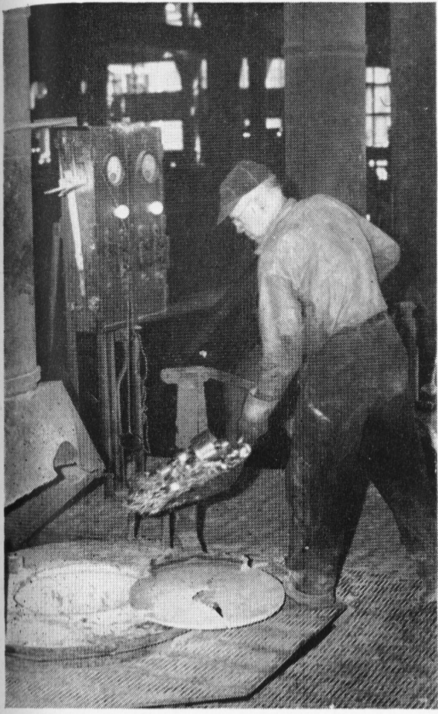
James Brennan, veteran employee in the Casting shop, is shoveling scrap into an electric melting furnace. A number of such furnaces feed the casting machine.
